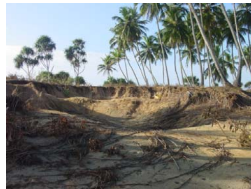
Severe erosion in coconut plantation at beach front
